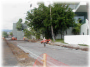
Fire Lane Construction
